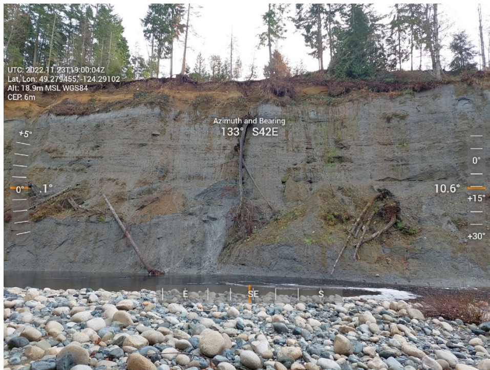
Photo 3.1 Photograph of the upstream eroding claybank (RK 8.6).
