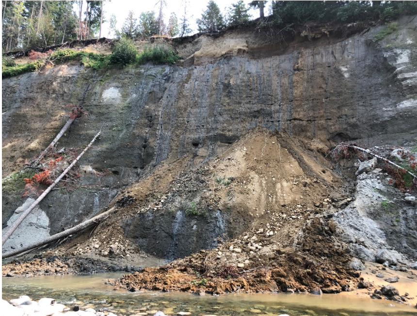
Photo 3.7 A slope failure occurred on August 26/27, 2023 during a dry, low flow period (Photo credit: Mid Vancouver Island Enhancement Society).
