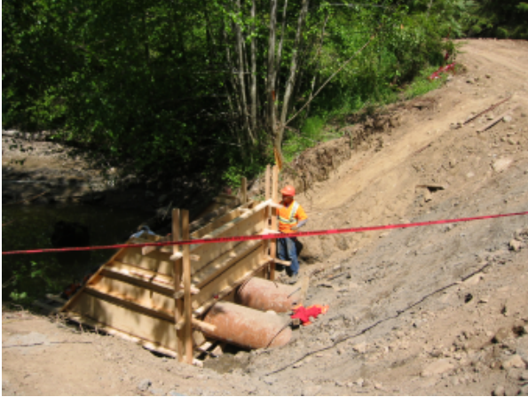
Figure 2 – Trash Rack Formed
