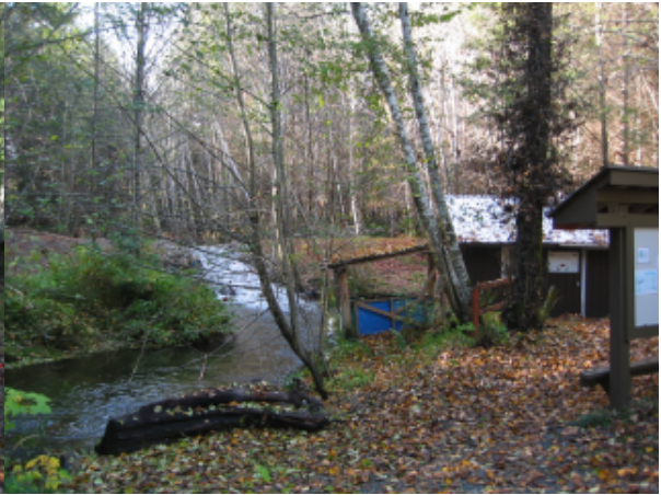
Figure 15 Newbury Weir Downstream
