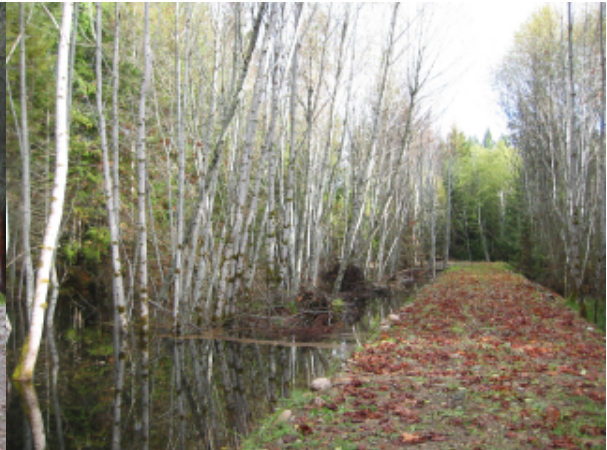
Figure 7 Completed Dyke - Beaver Pond
