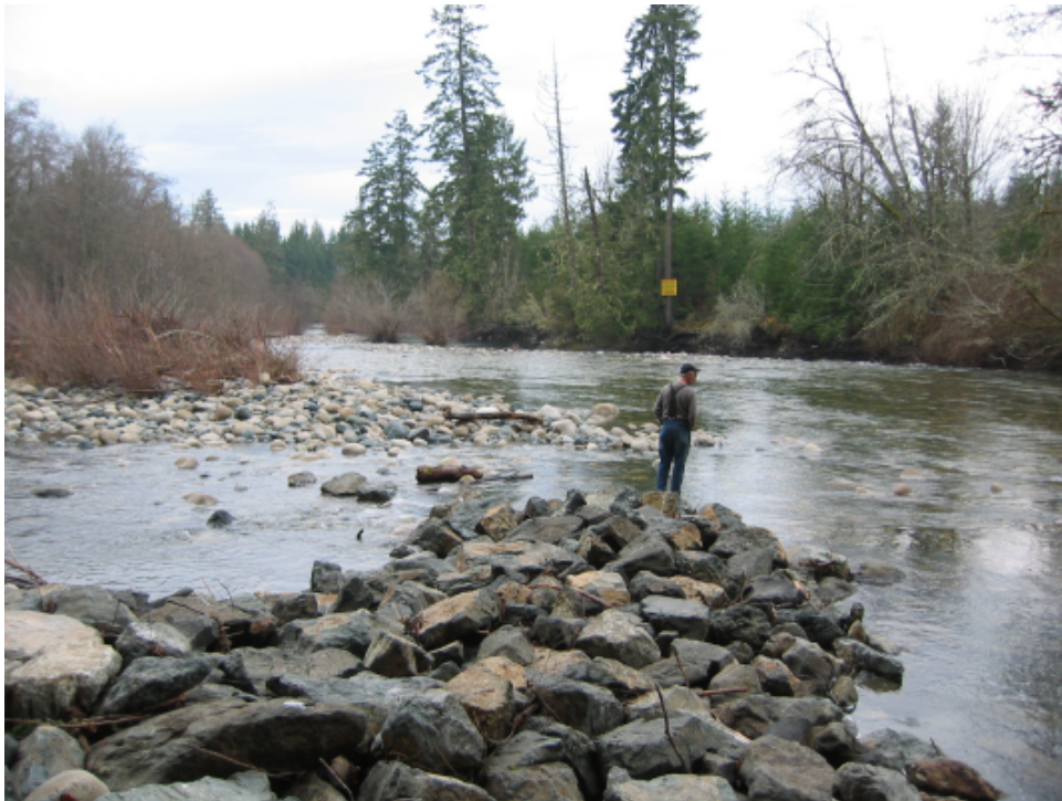
Figure 18 Flood Protection Groyne
