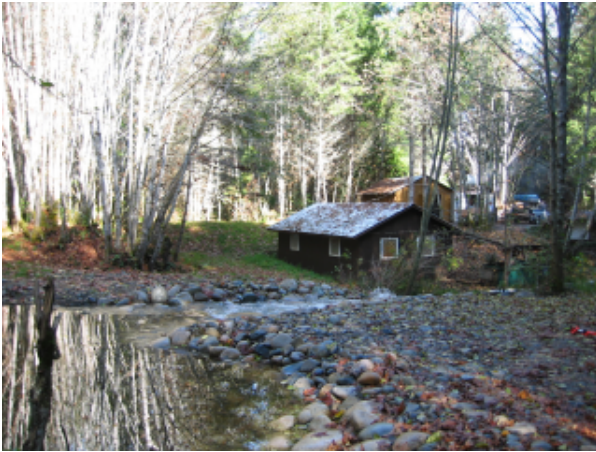
Figure 14 Newbury Weir Upstream
