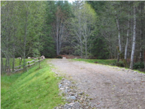
Figure 6 Completed Dyke – Settling Pond
