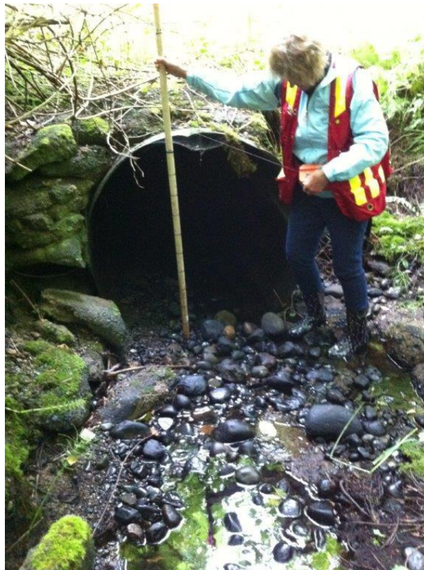
Figure 3. Measuring Cluvert at Blower Road
