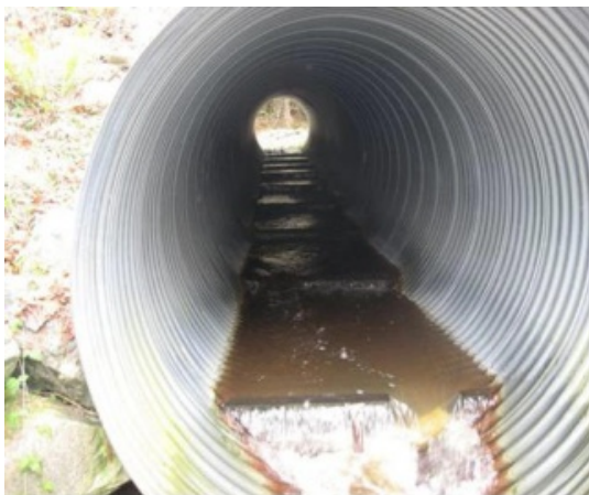
SHELLY CREEK: Baffled culvert and sediment retention pond installed under and adjacent to Wildgreen Way, respectively. Important steps in preserving healthy streams and fish populations.
