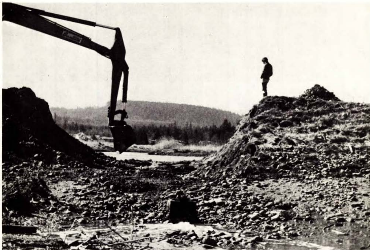
PLATE 2: Breaching the dyke at low tide, March 27, 1979
