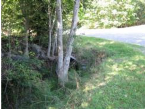
Enos Creek (S1) at Swallow Rd and Dolphin Drive looking upstream at 1,500 mm dia
