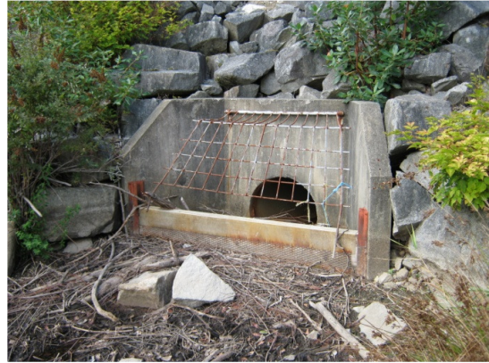
Enos Lake Outlet Structure
