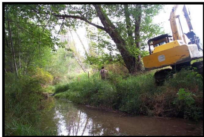
Morison Creek: Restoration Project
